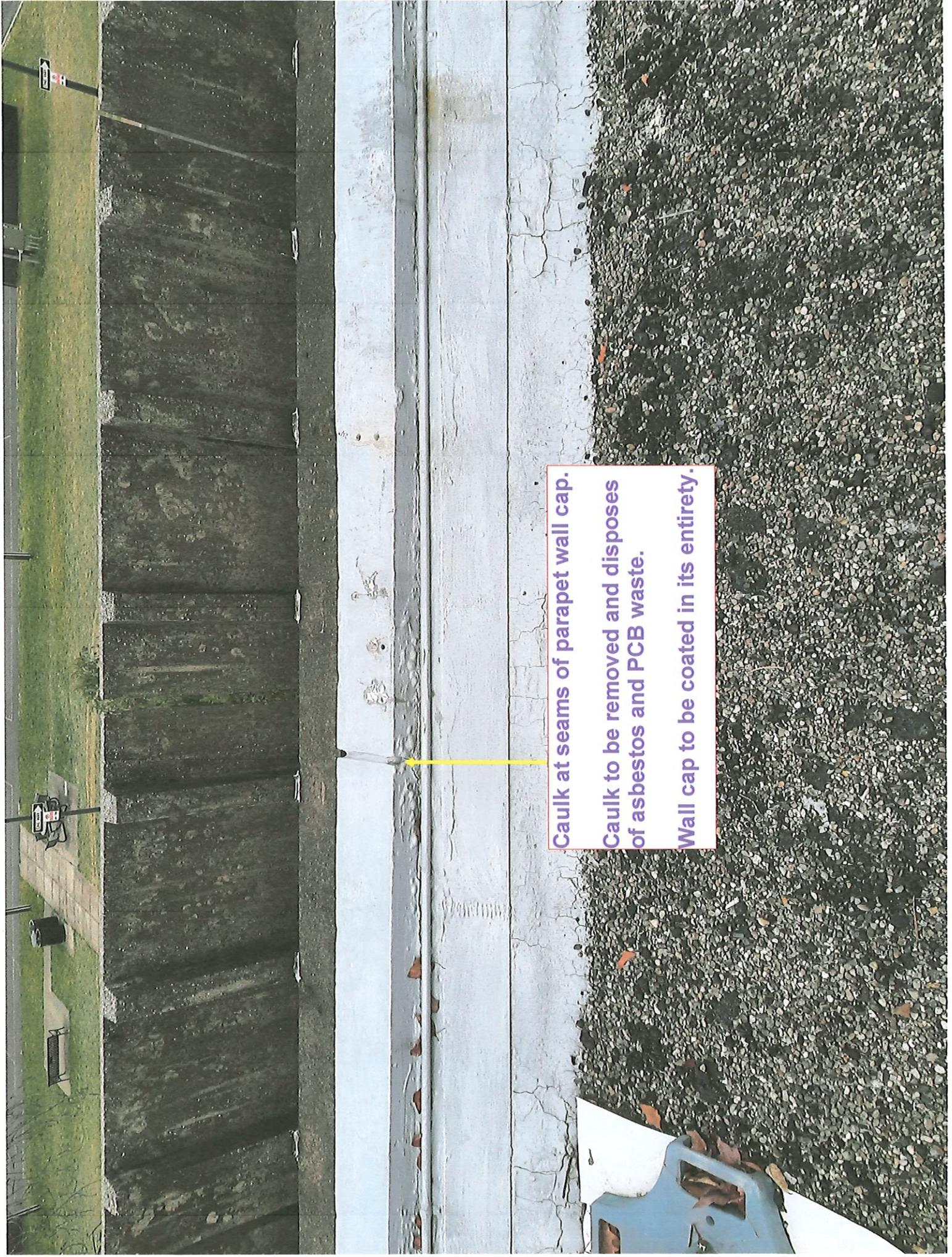
Caulk at seams of parapet wall cap.
