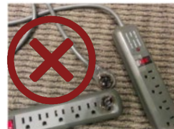
Do not group gang/overload power strips
