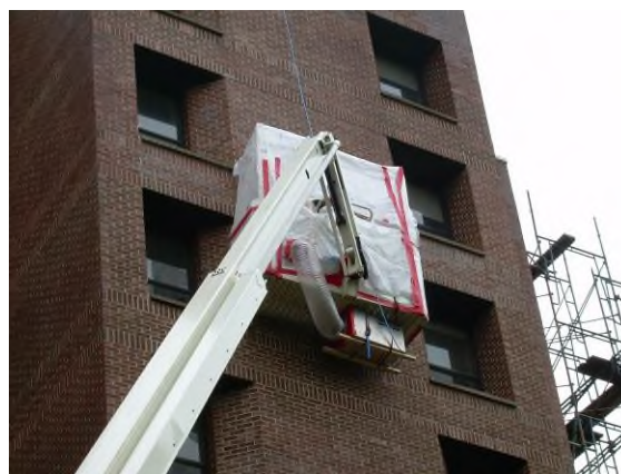
Polyethylene Containment on Boom Lift
