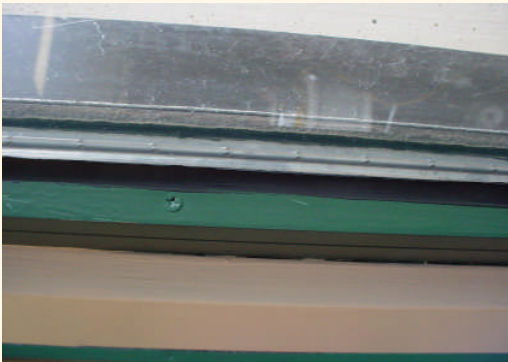
New caulking over existing glazing sealant
