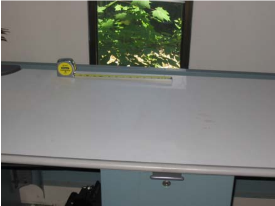
Photograph C.1 Room A-155, Sample 83945
