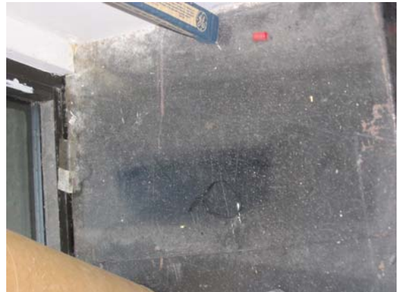
Photograph C.4 Room A-155, Sample 83948
