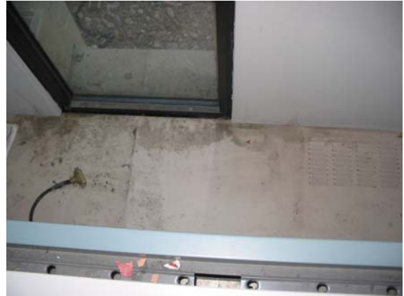
Photograph C.2 Room A-155, Sample 83946
