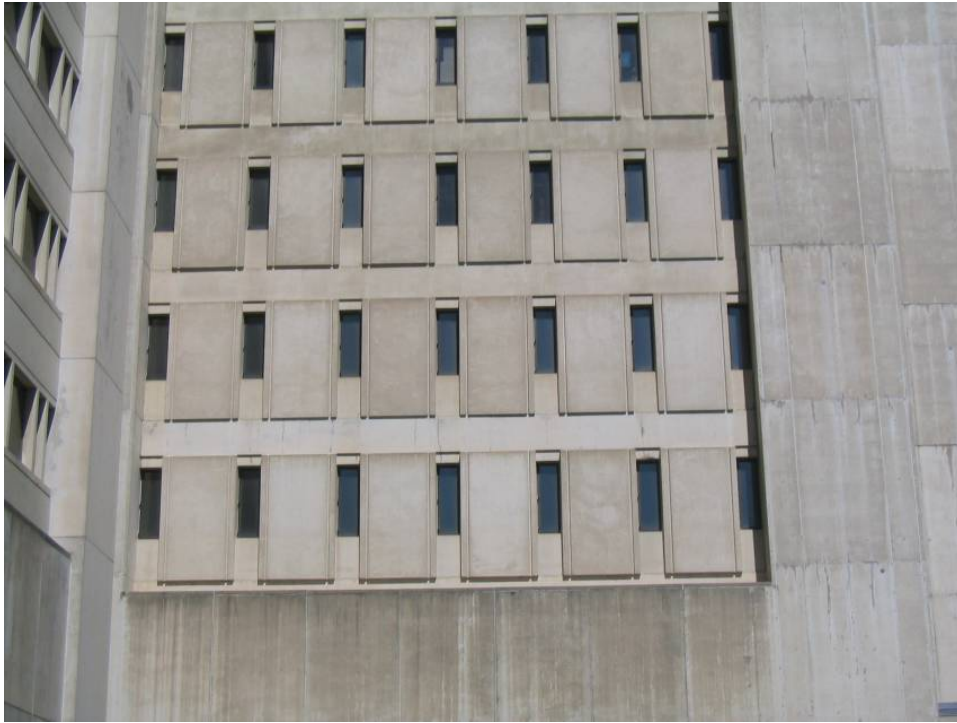
Photograph 1 Overview of South Elevation of Tower A
