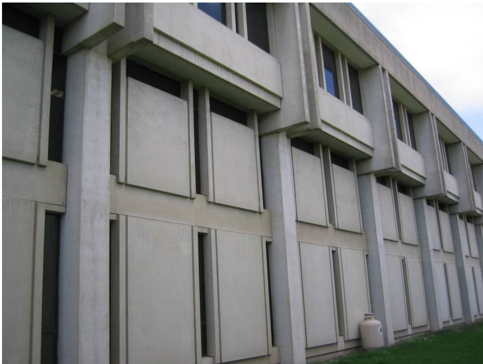
Photograph 2 Overview of North Elevation of Low-Rise Building
